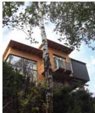
Simpson & Brown Architects have designed an innovative, low energy house in Currie that is super-insulated, air-tight and incorporates a mix of renewables. It is compact to minimise heat loss. A heat recovery system stores heat generated by occupants' cooking and showering for supply when required. Lifetime standards were adopted to allow for future adaptation with regard to accessibility.
